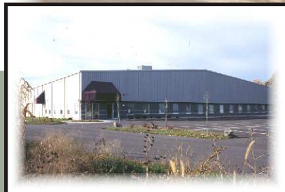
Pro-Tech Engineering; TJK Design & Const. Co., Inc., builder and architect.
