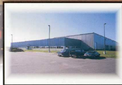
Pilot Industries; F.E.D. Corporation, builder; L.F. Sales & Engineering, engineer.
