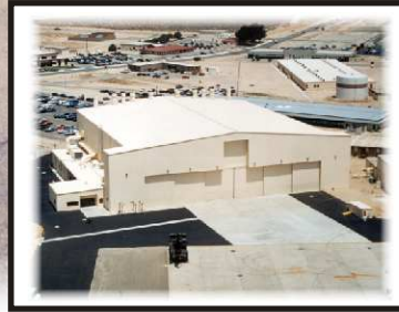
Corrosion Control Facility, Edwards Air Force Base; G and W Builders, Inc., builder.
