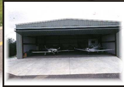
Halsey Hangar; D. G. Granade, Inc., builder.
