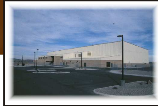
Above, Barstow-Daggett Heliport; G and W Builders, builder.
